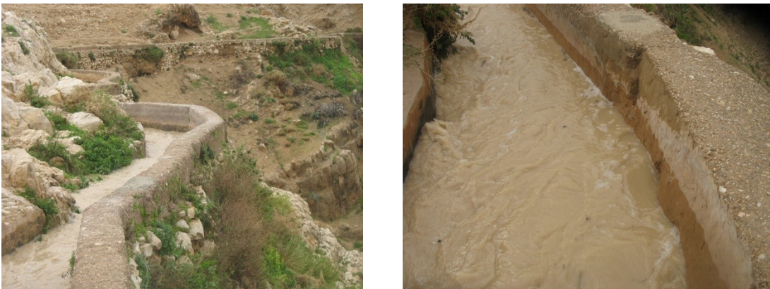
Figure 3.5: Highly turbid water transport in open canal at Aqbat Jaber.
